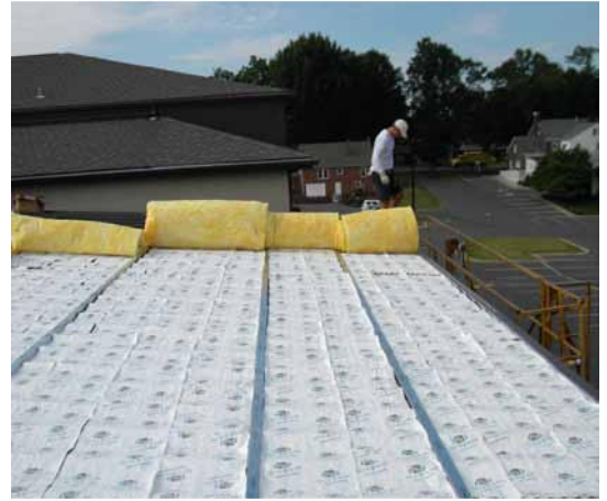
Retrofit onto an old roof.
