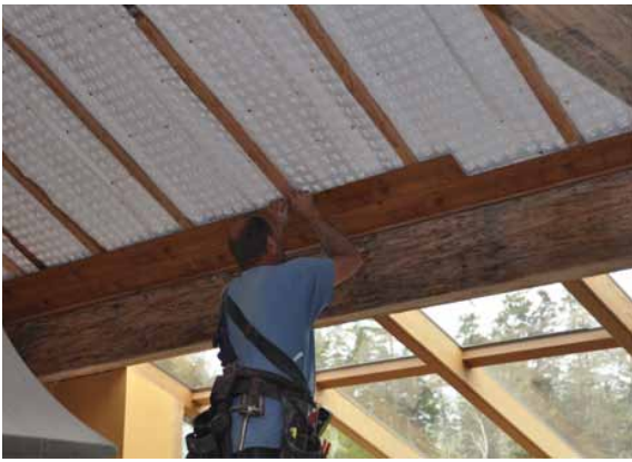
Attach to a ceiling before panelling.
